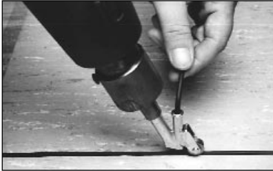
Figure 7: Forming center splice.
