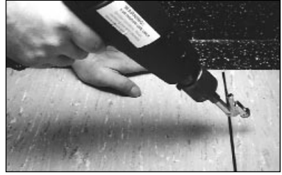
Figure 11: Glazing finishing weld.
